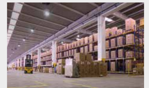
Lager und Logistik / Warehouses and logistics
